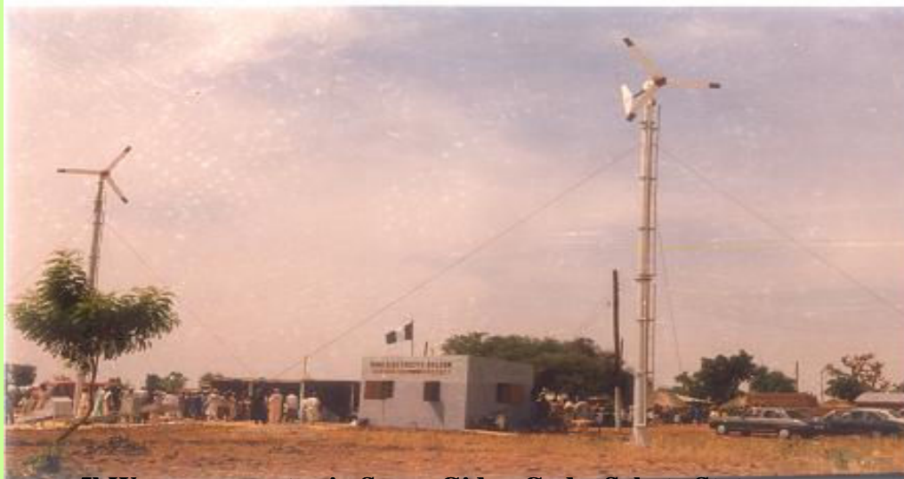
5kW aero generator in Sayya Gidan Gada, Sokoto State
